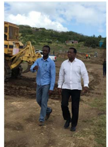
Hon. Eugene Hamilton on Site Visit at Cunningham Heights, Cayon
